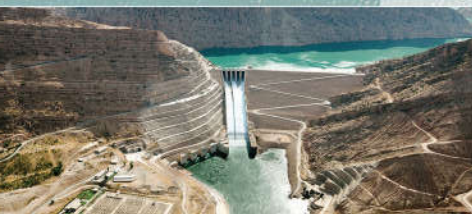
Masjed Soleyman Dam
